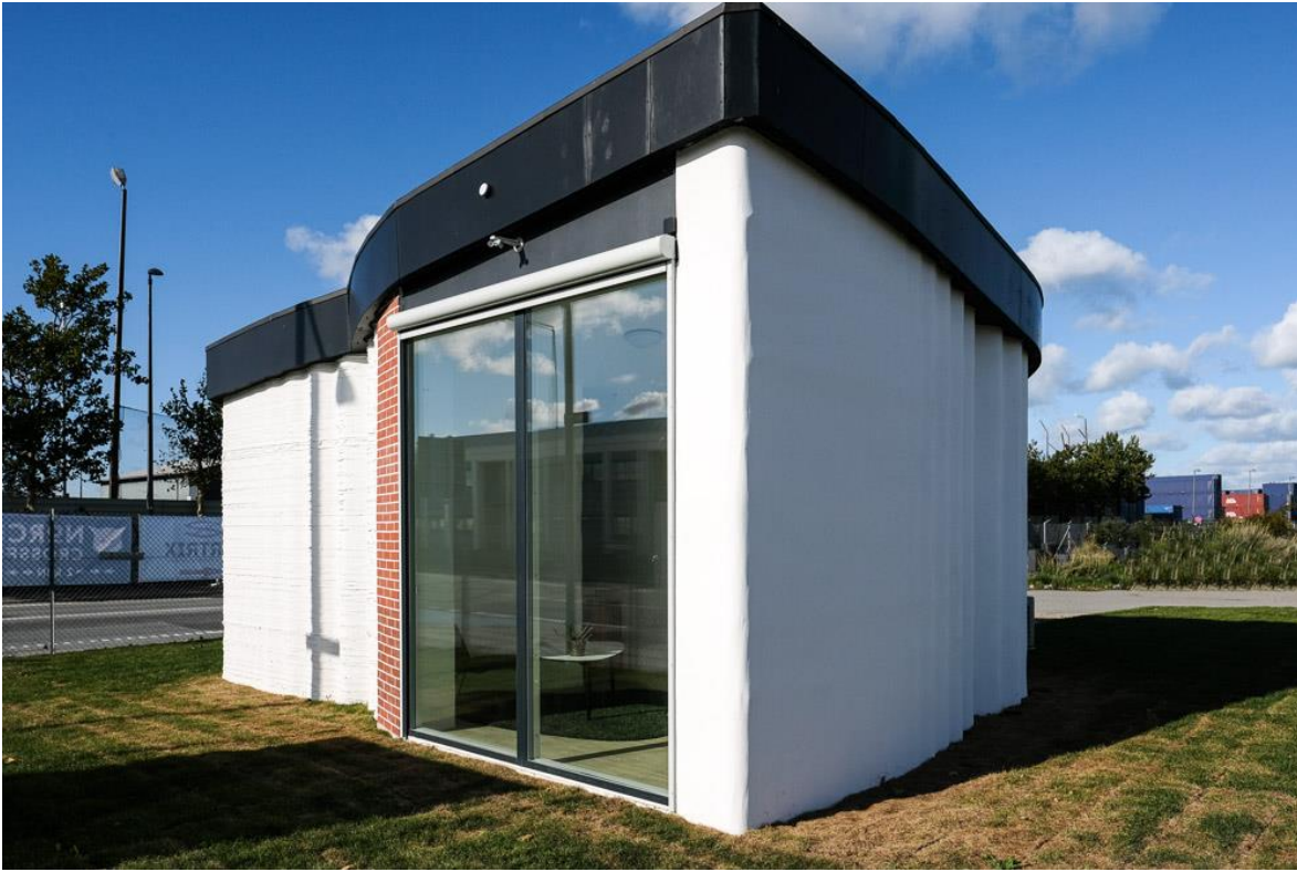
The BOD building in Copenhagen, Europe's first 3D printed building (Architect Ana Goidea, MAA)
