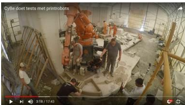
Person in black t-shirt removing excess material with spatula at point where the printer is printing a double corner (180 degree turn)
