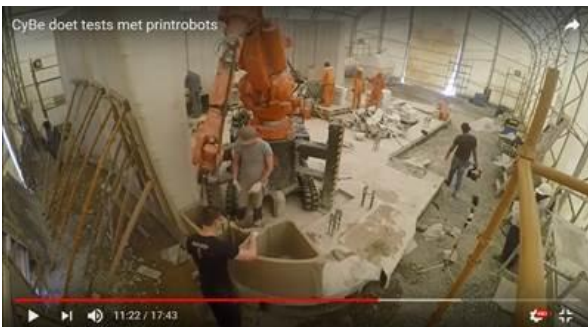
Print head tilting to reach the corner, needed due to sectional printing, but no bonding occurs between new and existing print
