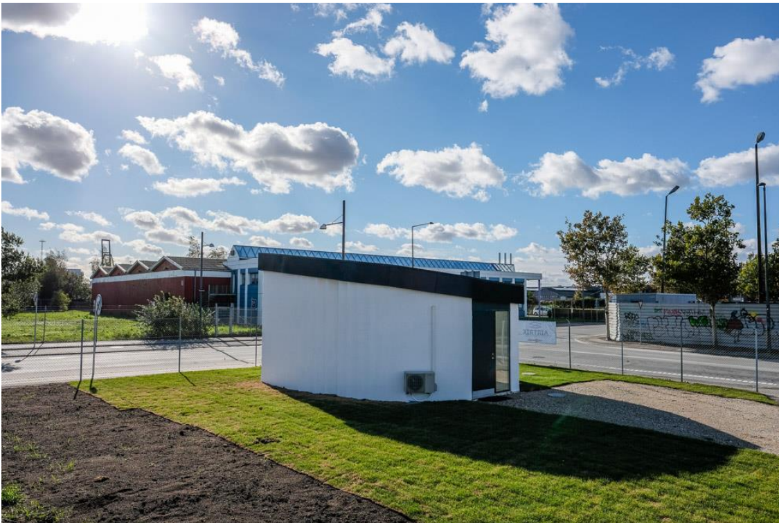
Picture of The BOD in Copenhagen, Europe's first 3D printed building, done by COBOD in the fall of 2017.
